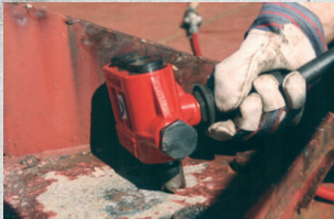
Thick Paint Removal
