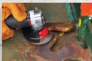
Weld Seam Removal
