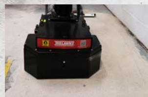
Polishing Concrete Floors
