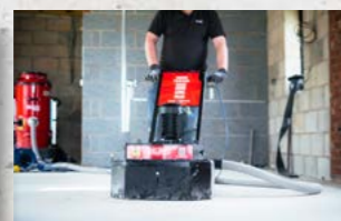
Removing High Spots
