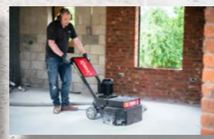
Grinding Concrete
