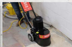
Grinding Concrete
