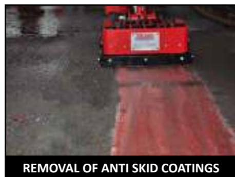
COATING & CORROSION REMOVAL
