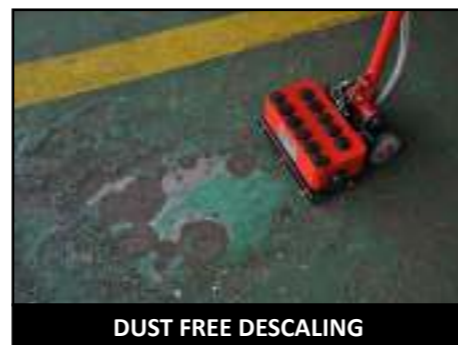
REMOVAL OF ANTI SKID COATINGS
