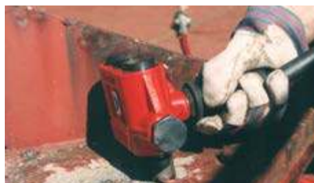
CORROSION REMOVAL
