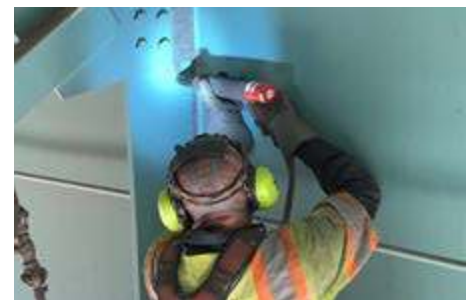
CORROSION REMOVAL
